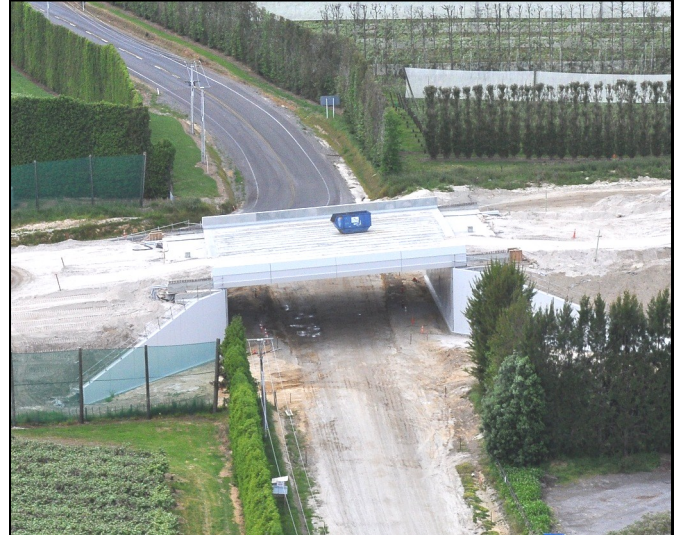
Below right: Maketu Road bridge
