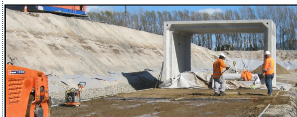
Left: Mowing Boat Culvert B
