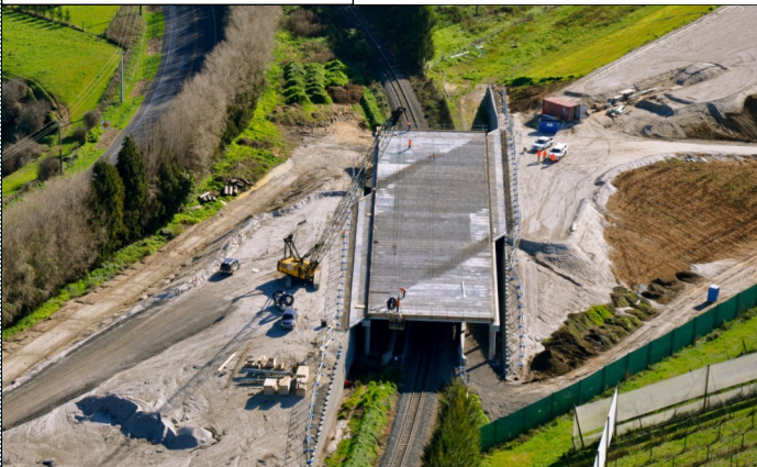
East Coast Main Trunk rail bridge
