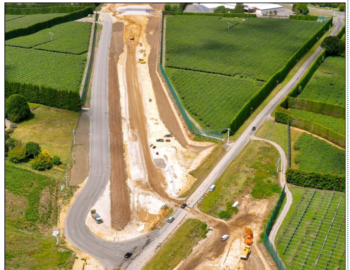
Above: The re-aligned Te Tumu Road, on the left.
