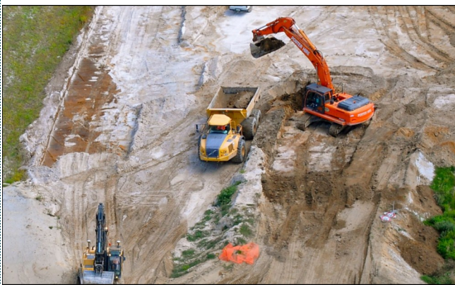
Above: Surcharge being removed between Domain Road and Parton Road
