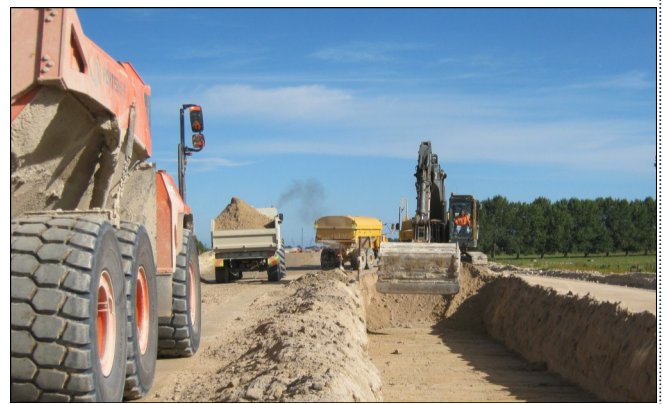
Above: Surcharge being removed near Pah Road
