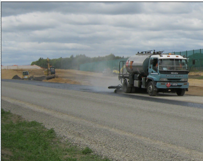
Above: Bitumen being sprayed prior to sealing chip being applied.
