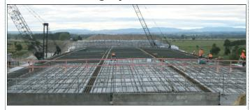
The last steel section is about to be lifted into place, which will complete the 186 metre bridge, which spans not just the river, but the future realigned Bell Road.
