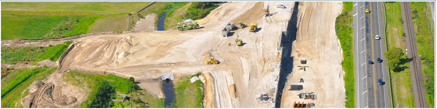
Maranui Drain culvert at the Mangatawa Interchange
