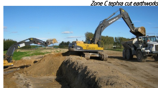
Zone C tephra cut earthworks
