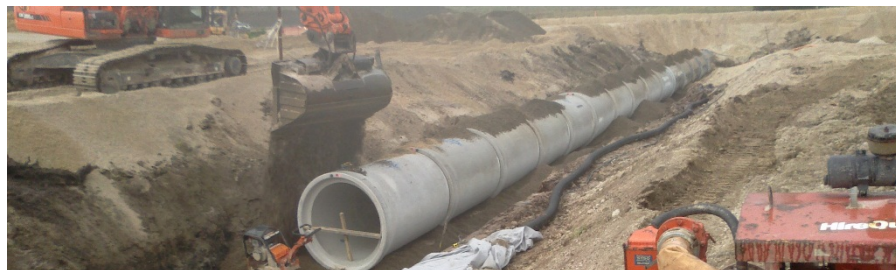
Left: The Zone C, 99 metre x 1350 millimetre culvert under construction
