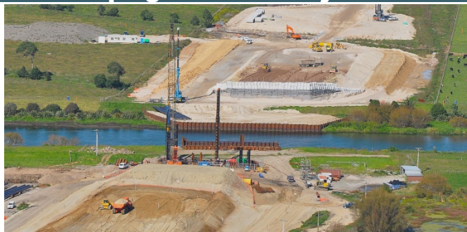
Kaituna River bridge abutments and Pier B piling operation
