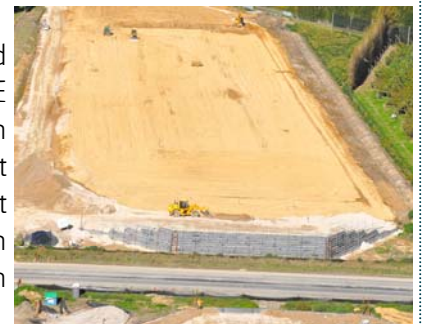
The Maketu Road bridge southern MSE wall
