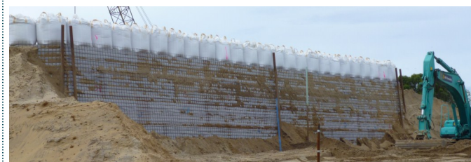
Kaituna River bridge west MSE wall
