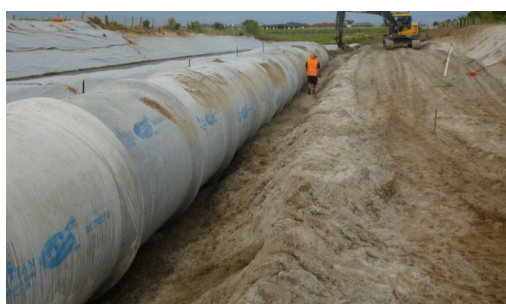
An 80 metre long, 2100mm diameter Maranui Drain culvert
