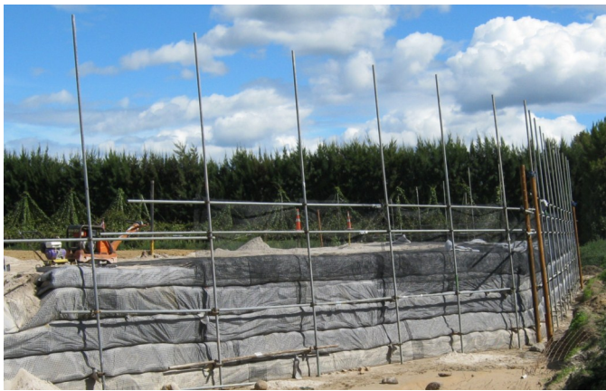
Above: Maketu Road bridge MSE wall under construction
