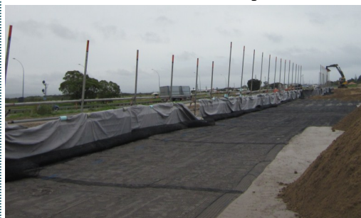
Mangatawa Interchange MSE wall (early March)
