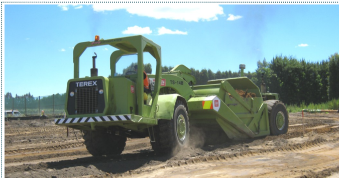
Topsoil stripping at the Maketu Road bridge site
