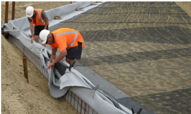
A 500mm layer being prepared with a steel mesh face
