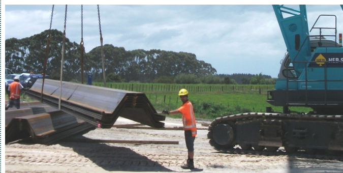
Sheet piles arrive at the Kaituna River bridge east site
