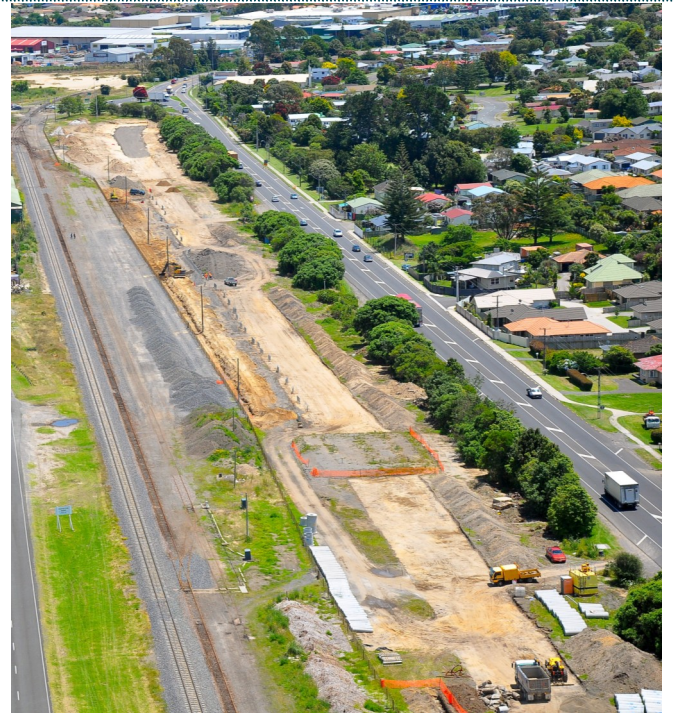
Te Maunga northbound lanes begin to take shape
