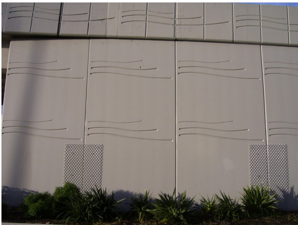
An example of concrete panels. These are on the Hewletts Road flyover
