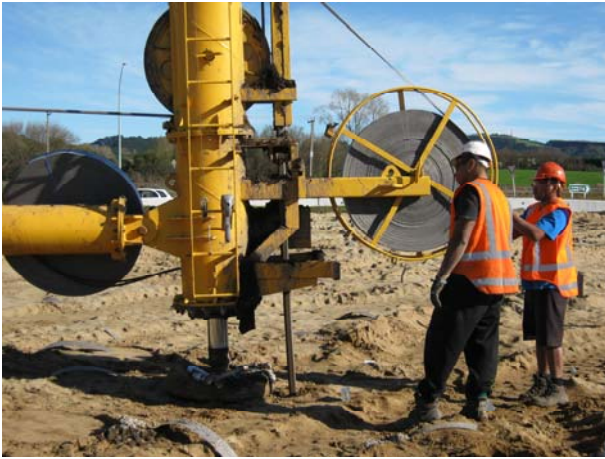
Wick drains being installed at the Domain Road interchange
