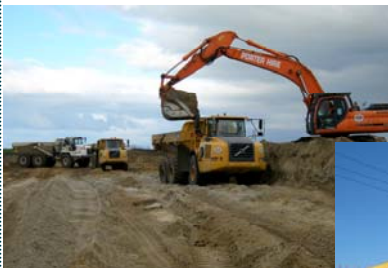
Left: Moxy's ready for loading at the sand cut
