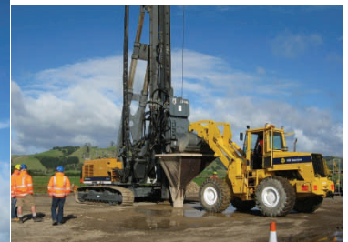
Stone column trials undertaken at the TEL Project Office, Tara Road
