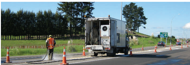
Domain Road lane re-alignment underway
