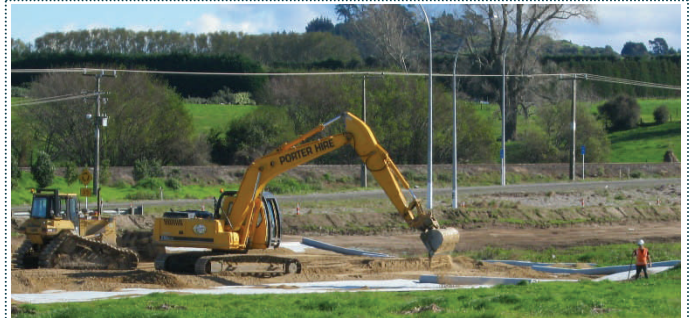
A sand blanket under construction at Domain Road
