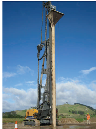
Stone column trials undertaken at the TEL Project Office, Tara Road
