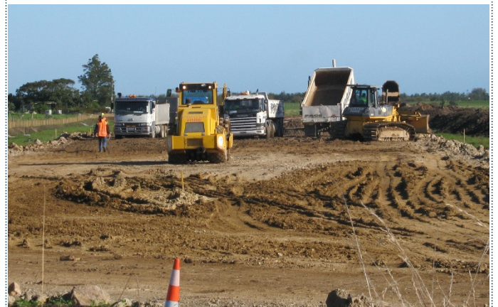
Pah Road haul road under construction - view toward Kaituna River
