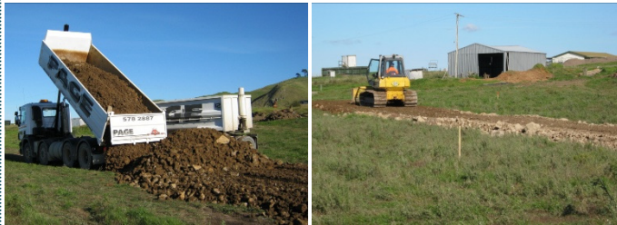
Domain Road haul road underway
