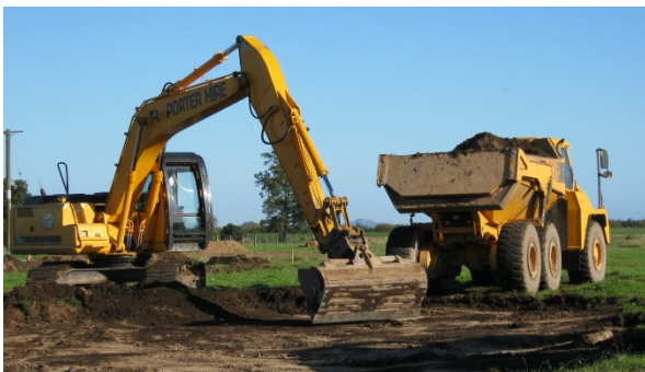
Topsoil stripping in preparation for the haul road material
