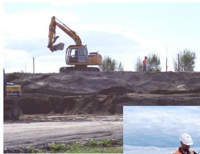
Pah Road trial embankment
