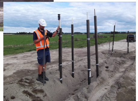
Monitoring the equipment installed in the trial embankment
