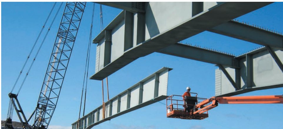
Kaituna River bridge and Bell Road 2014
