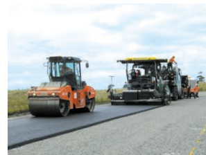
Asphaltic concrete being paved over chipseal (Type A )
