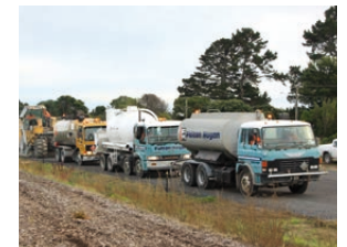
Foamed bitumen stabilisation of the base layer (Type B )
