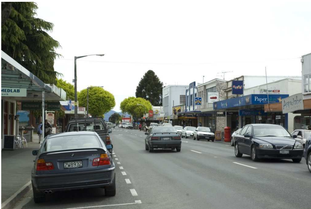
High Street (SH60) Motueka, viewed towards the north
