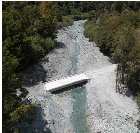
After the completion of repairs
