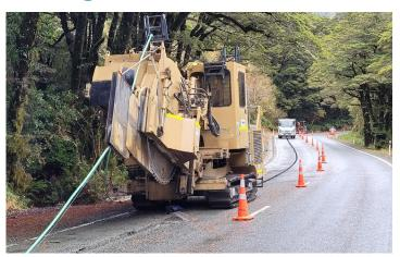
Crews laying fibre optic cable on State Highway 94 between Te Anau and Milford Sound have reached the alpine area near Monkey Creek on the eastern side of the Homer Tunnel. This fibre will transform telecommunications between Te Anau and Milford Sound enabling greater use of communications technology including cell phones and high-speed internet access for the businesses at Milford Sound. With less traffic using the highway, it's an ideal time to install this technology.
