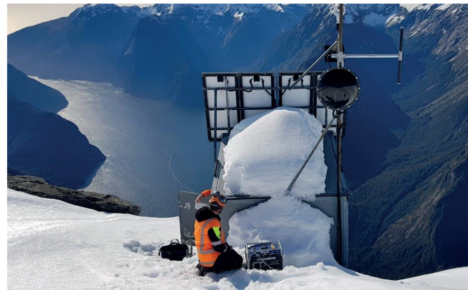
Weather station maintenance underway on a station located high above Milford Sound.
