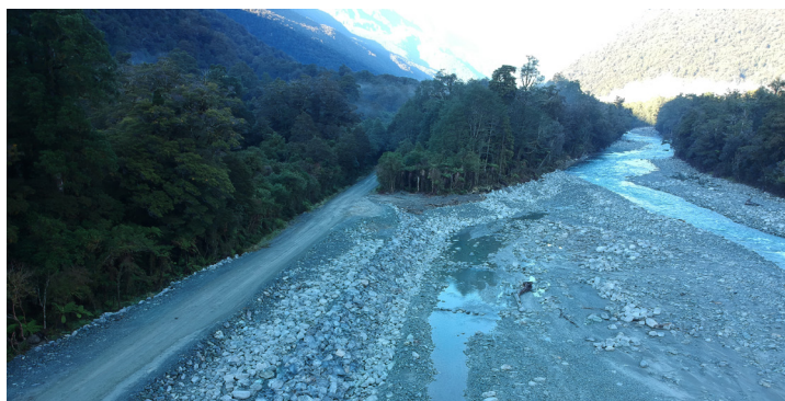
A repaired section of the Hollyford Road
