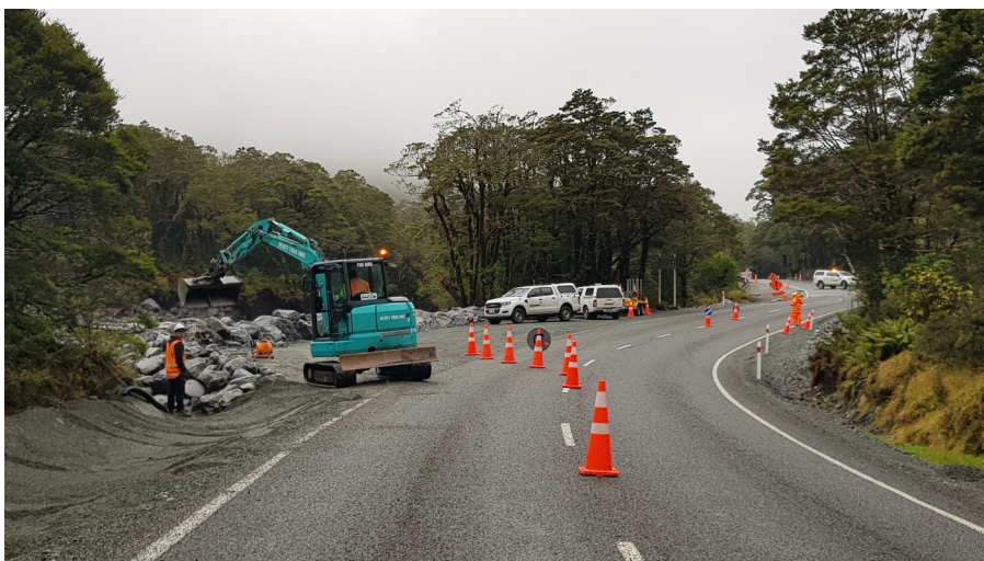
Storm reconstruction work underway at Windfall Creek.
