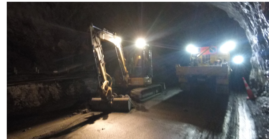
Road surface repairs in the Homer Tunnel.
