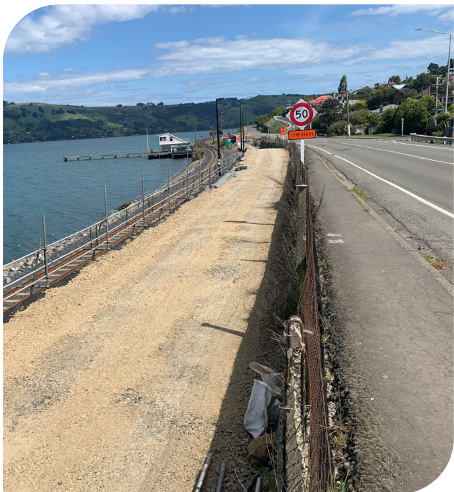
Mechanically stabilised earth retaining wall at St Leonards
