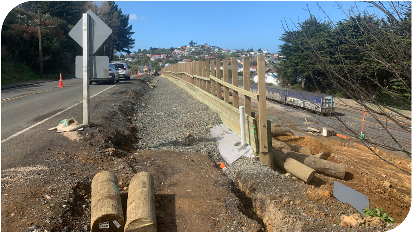
Large timber retaining wall at Port Chalmers
