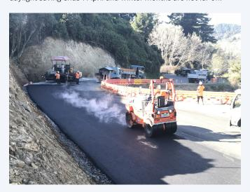
Laying asphalt on one of the feshly widened corners, in preparation for truck and trailer units on Tuesday.
