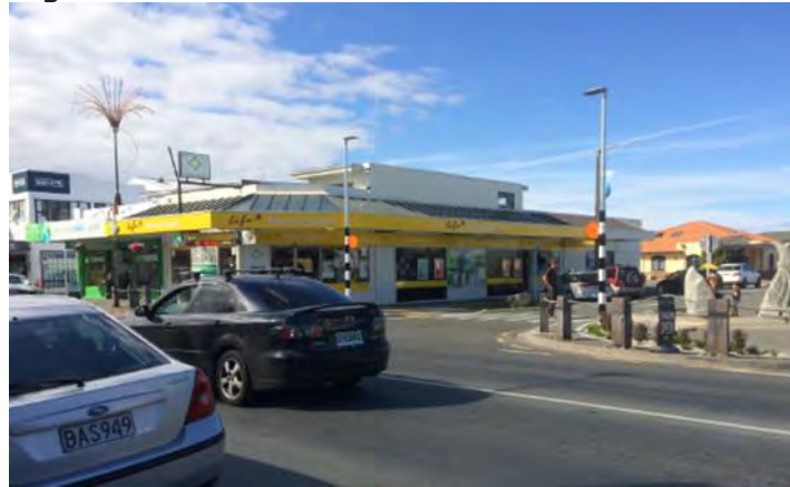
Site 4: Zebra crossing on Wallace Street close to High Street intersection.
