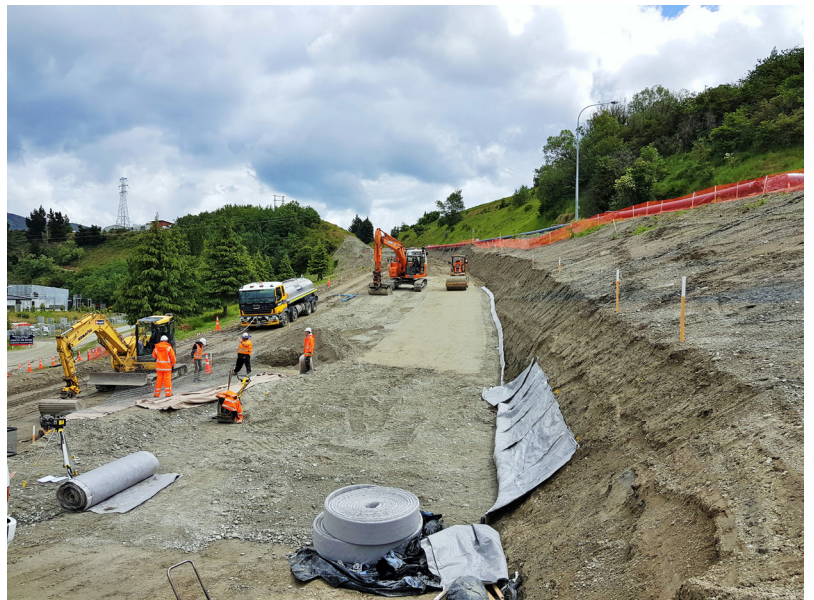
The new slip road worksite looking towards Frankton
