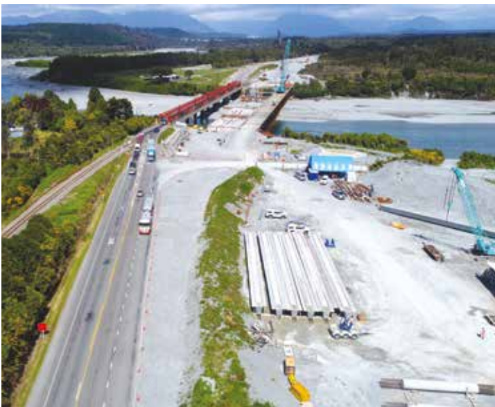
Work on the new road alignment is going well
