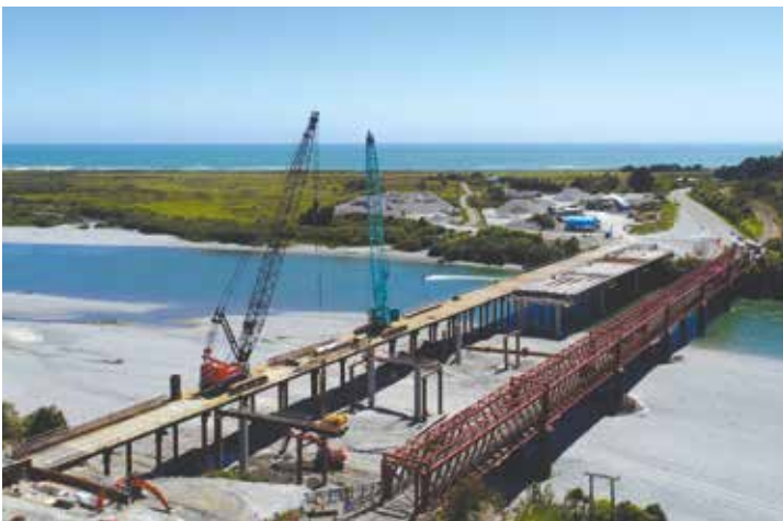
The new Taramakau Bridge is taking shape
