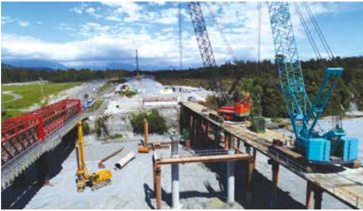
Working in the river bed
