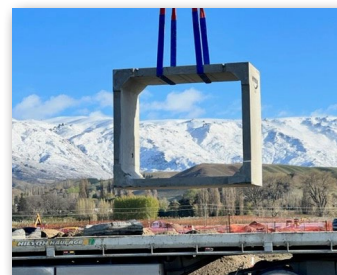
Above: A section of the underpass being lowered in place.
