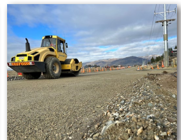
Above: The road being built on SH6 near McNab Road.
