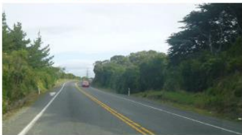
Example of SH58 before improvements
