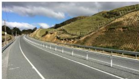
Example of SH58 after improvements
