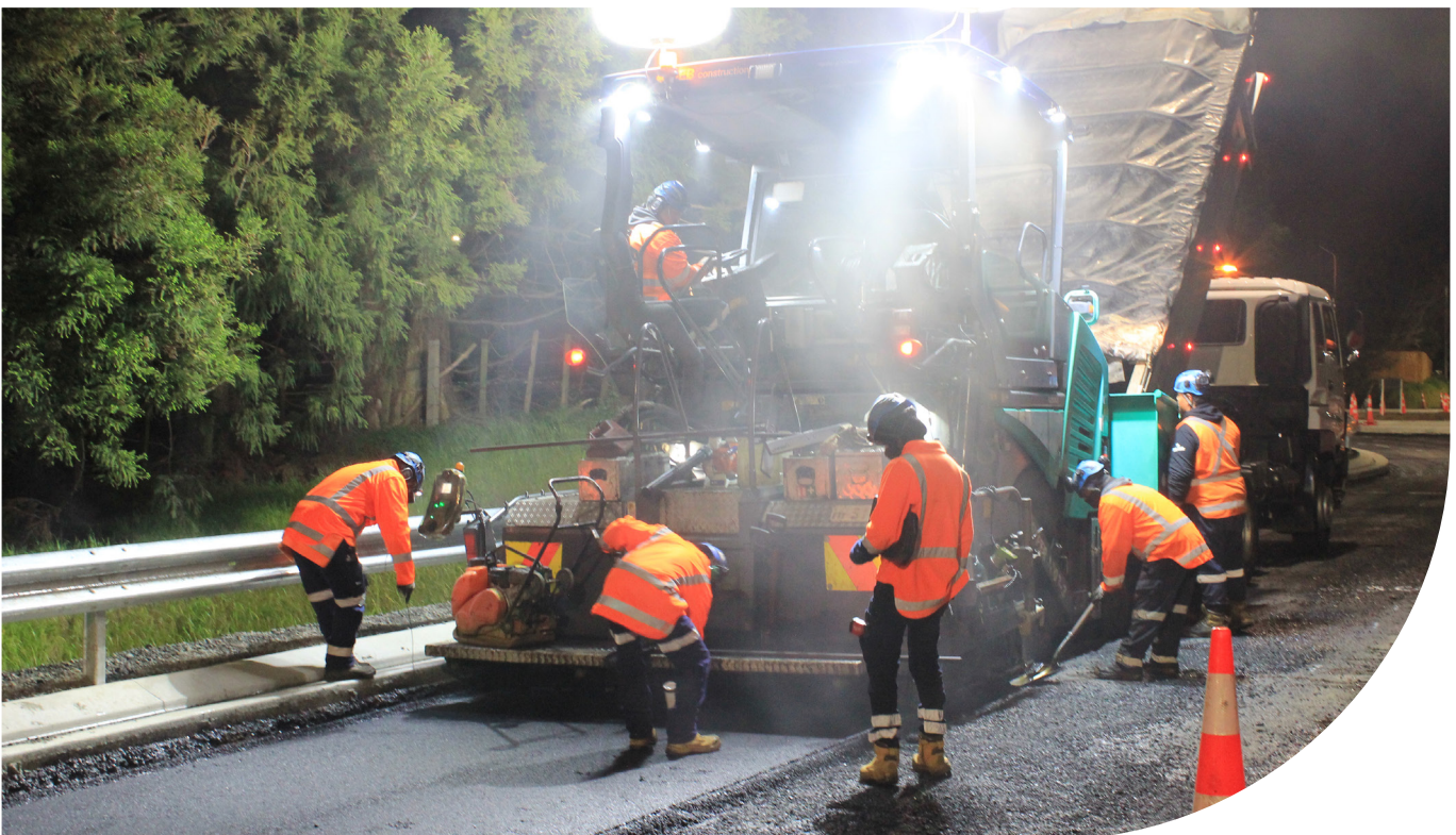
Night work in progress at SH2 / Rea / Tetley roads
