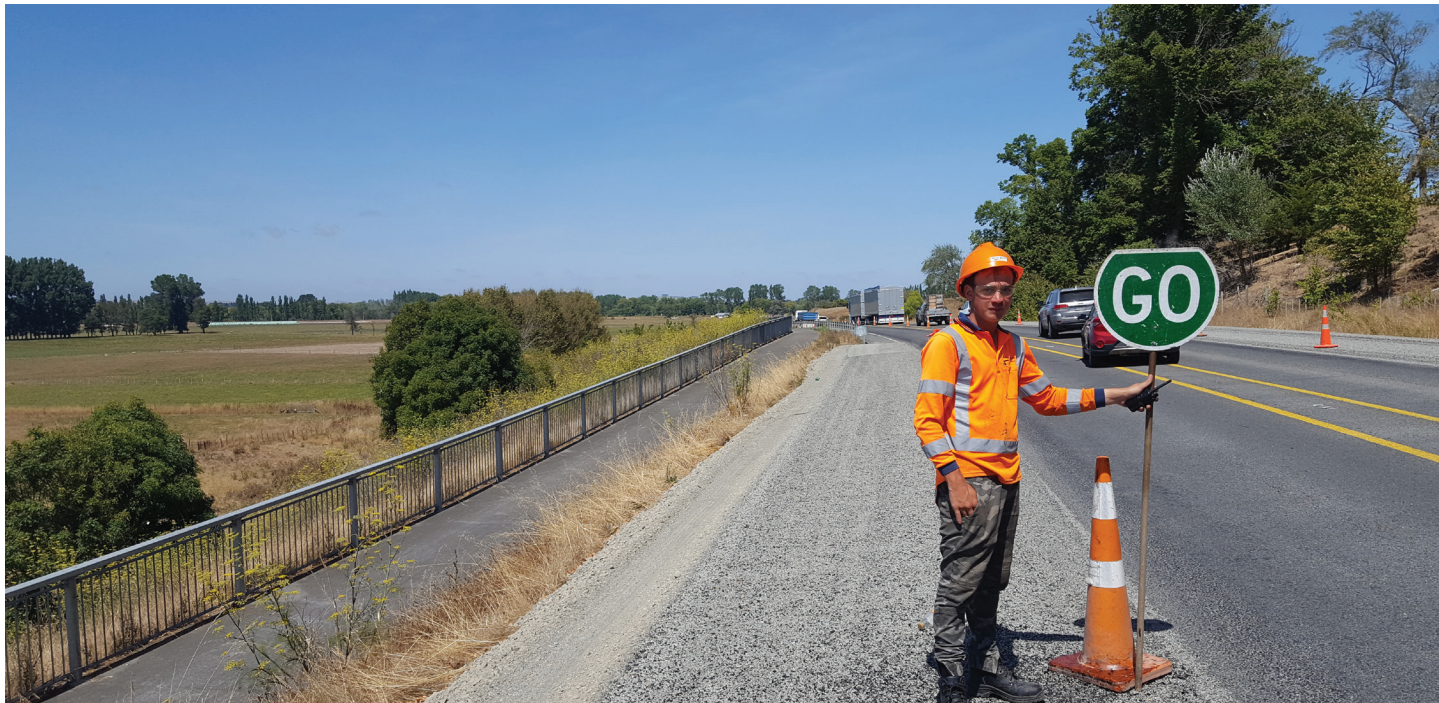
Road widening prior to installing barriers between Waipukurau and Waipawa.
