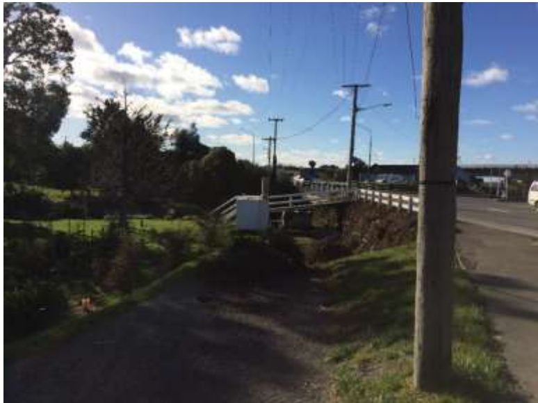
Figure 12: View of the northern side of State Highway 1 at the Lyell Stream Bridge.
