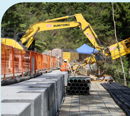
Slip A3 - Anchors being installed.
