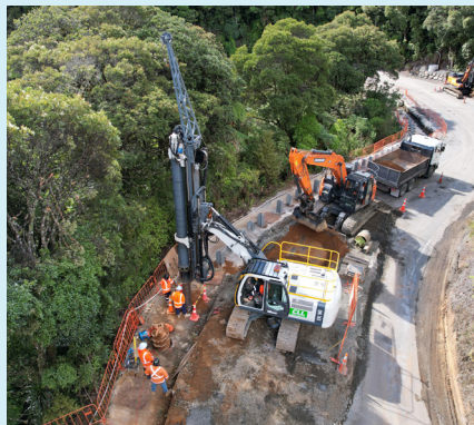
Slip A26 - UC Piling rig in action.
