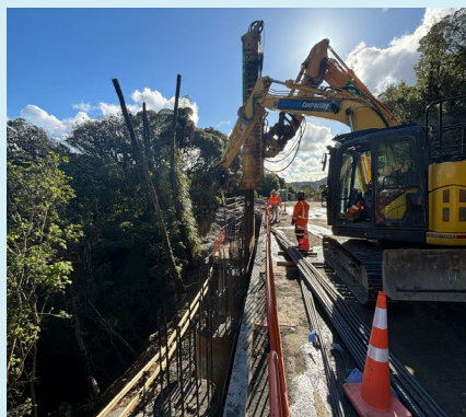
Slip A6 - Driving the lagging plates behind the permanent piles.
