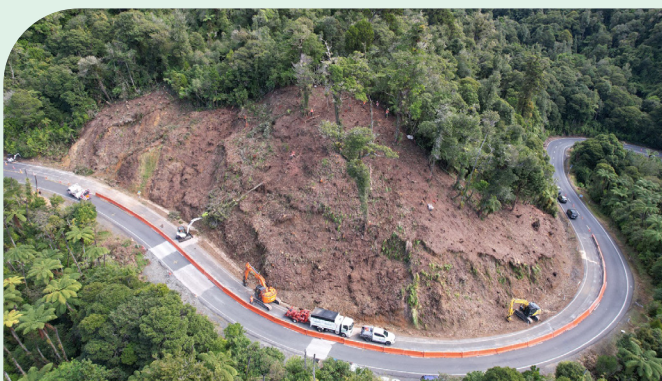
Progress with the clearing of vegetation and beginning of earthworks on A11 (left photo taken 30 April 2024, right photo taken 14 May 2024). All land and vegetation is carefully checked and wildlife relocated prior to anything being removed.
