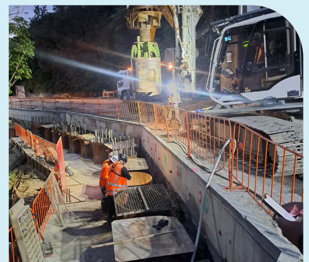
Slip A6 - Piling during night works.
