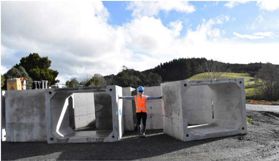
Fulton Hogan's Stakeholder Manager, Mel Norris, stands next to sections of the new concrete box culvert. Each 2m section weighs 4.7 tonne.
