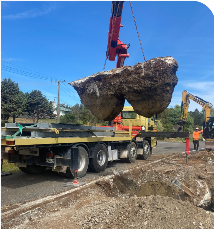
Removal of the old traffic island.
