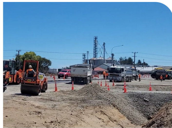
Turnaround facility construction site.
