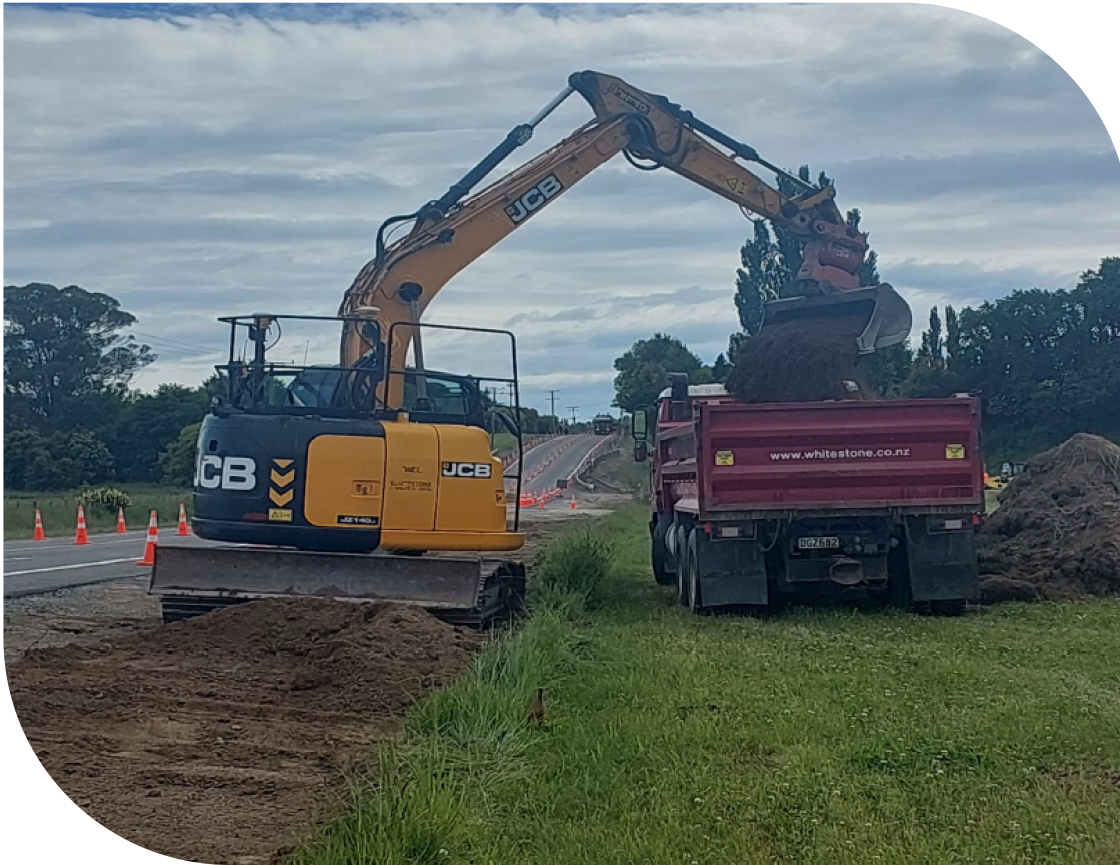
Site clearance work at the northern end of the project area.
