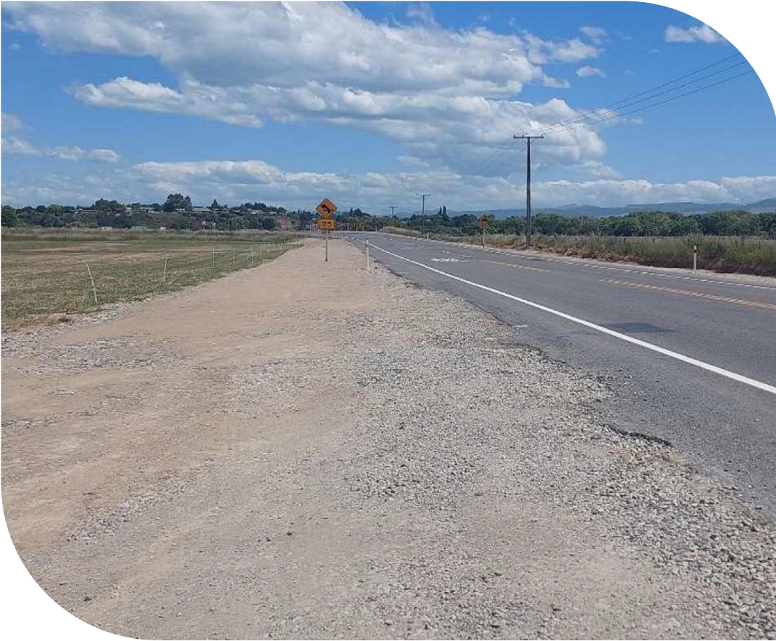
On site highway road shoulder work looking south toward Maheno.
