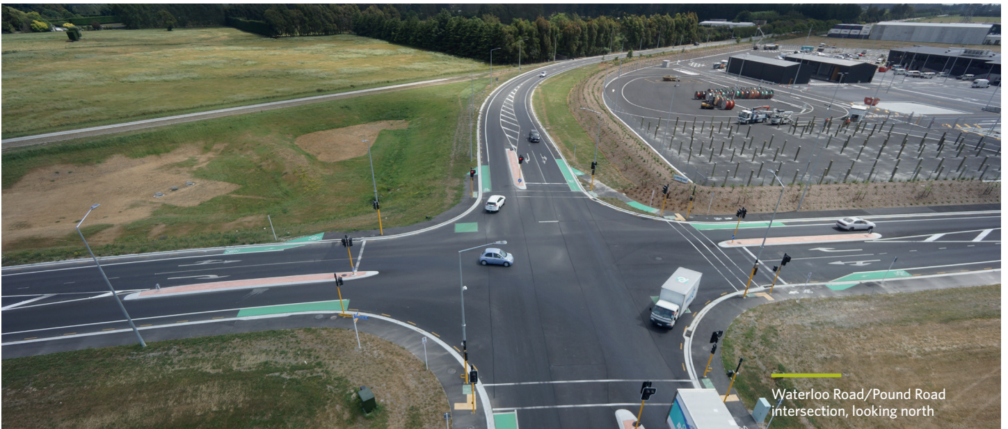
Main South Road (SH1)/Pound Road intersection, looking north
