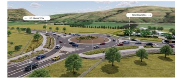
The Howards Drive roundabout will make this intersection safer. Safety concerns have seen this T-intersection prioritised because the speed through this area is higher and is currently controlled by a give way sign. The roundabout will be similar to those at Stalker Road, Hawthorne Drive and Grant Road. Better access to the Ladies Mile Pet Lodge will be provided from the north side of the roundabout.
