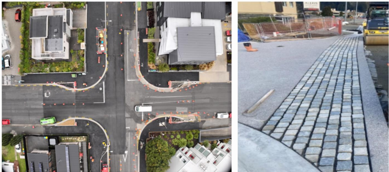
Above left, new footpaths at the Sydney and Melbourne Street intersection, and right, cobblestone pavers laid on Frankton Road. Work is already underway to install flush crossings and pavers on upper Suburb Street. Once this is reopened, the focus will shift to installing flush crossings and pavers on Dublin Street.
