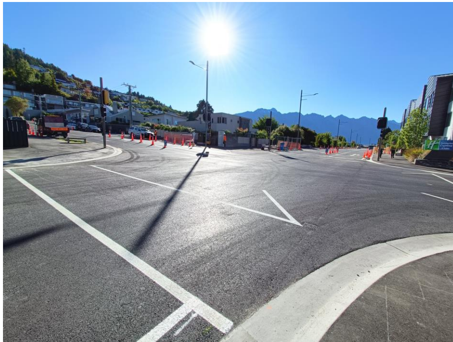
Ready for traffic...the intersection of Sydney and Melbourne Streets.
