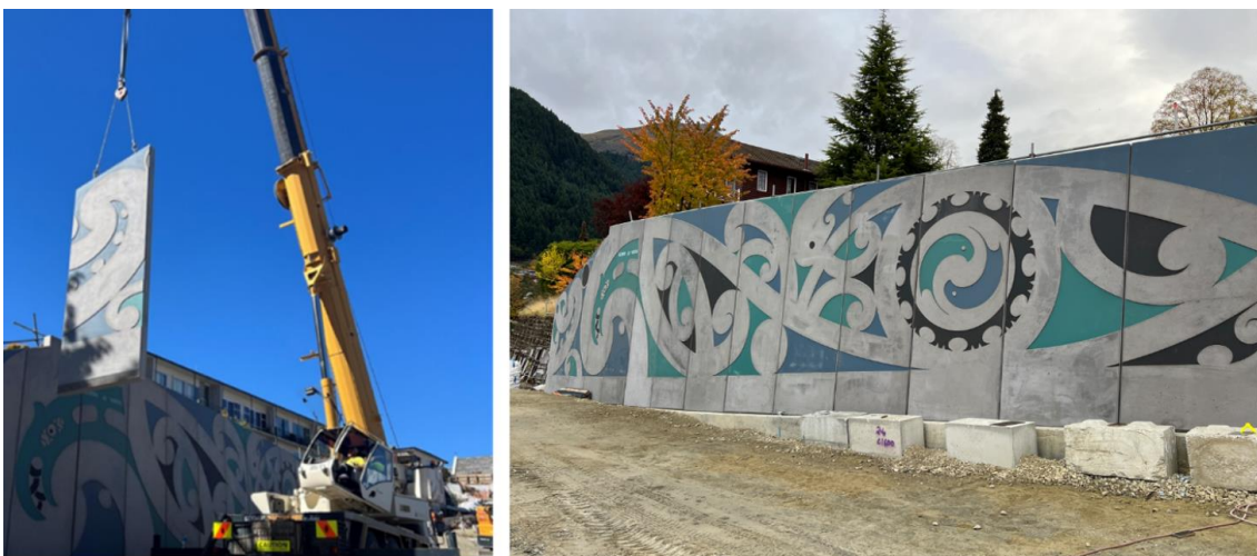
The Ballarat Street precast concrete panels were installed with millimetre-precision.
