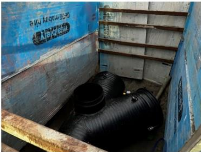
Large trenches are needed for the new 1.4m diameter stormwater pipes.
