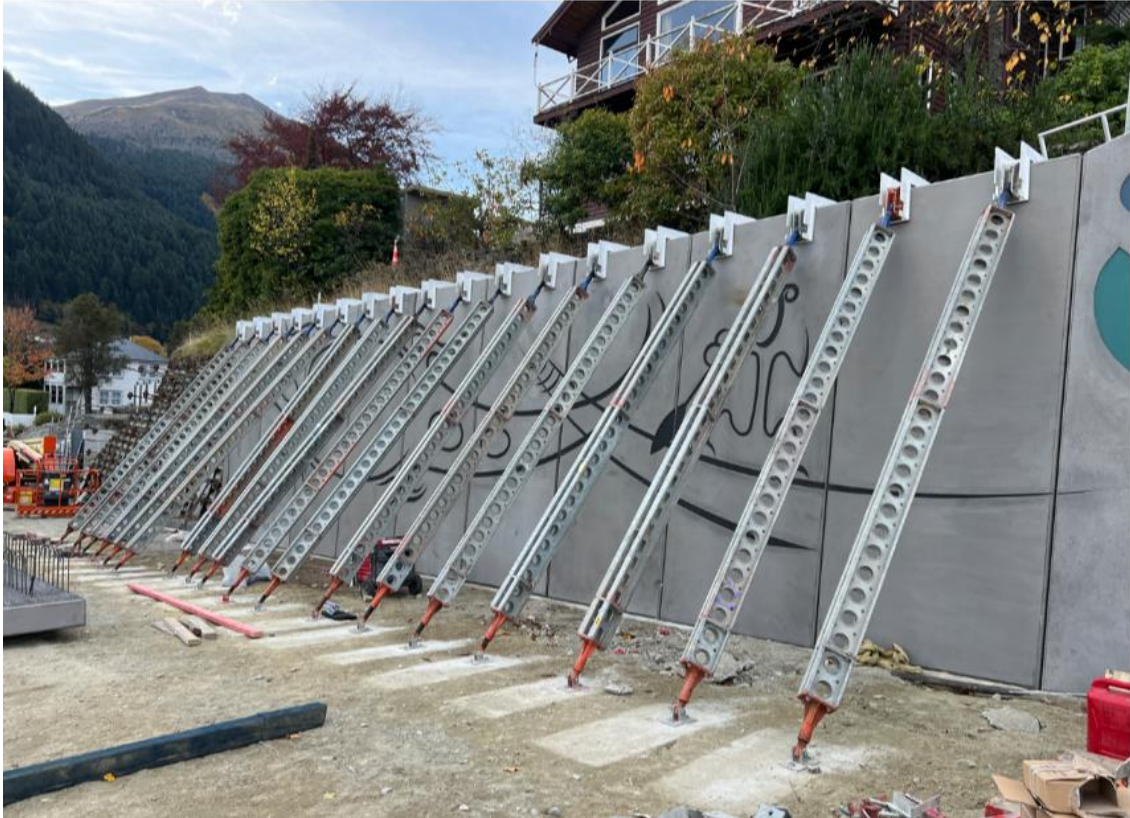
Some of the 58 large decorative panels being installed along Henry Street.
