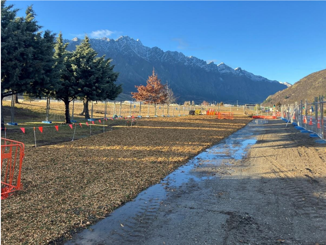
Neat, tidy and protected... the newly-covered trench along SH6 Kawarau Road.
