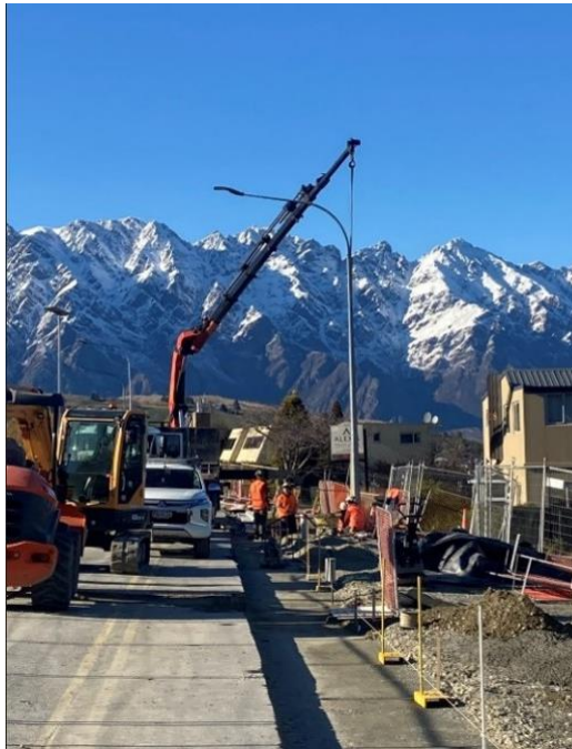
A bluebird day for light pole installation on Frankton Road.
