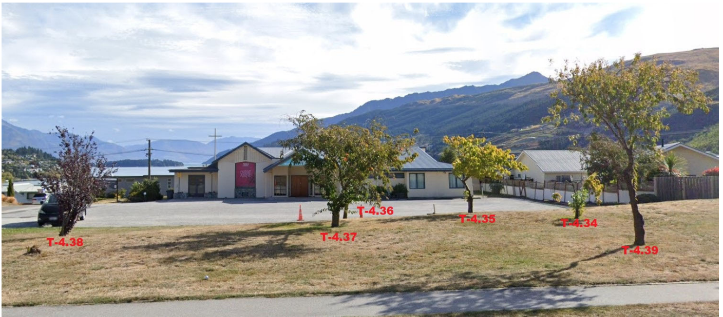
Photo – western side of SH6 corner with Ross St.
