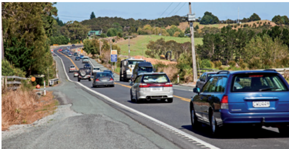
The Puhoi to Wellsford highway project will address congestion issues which are a common complaint of the current SH1.
