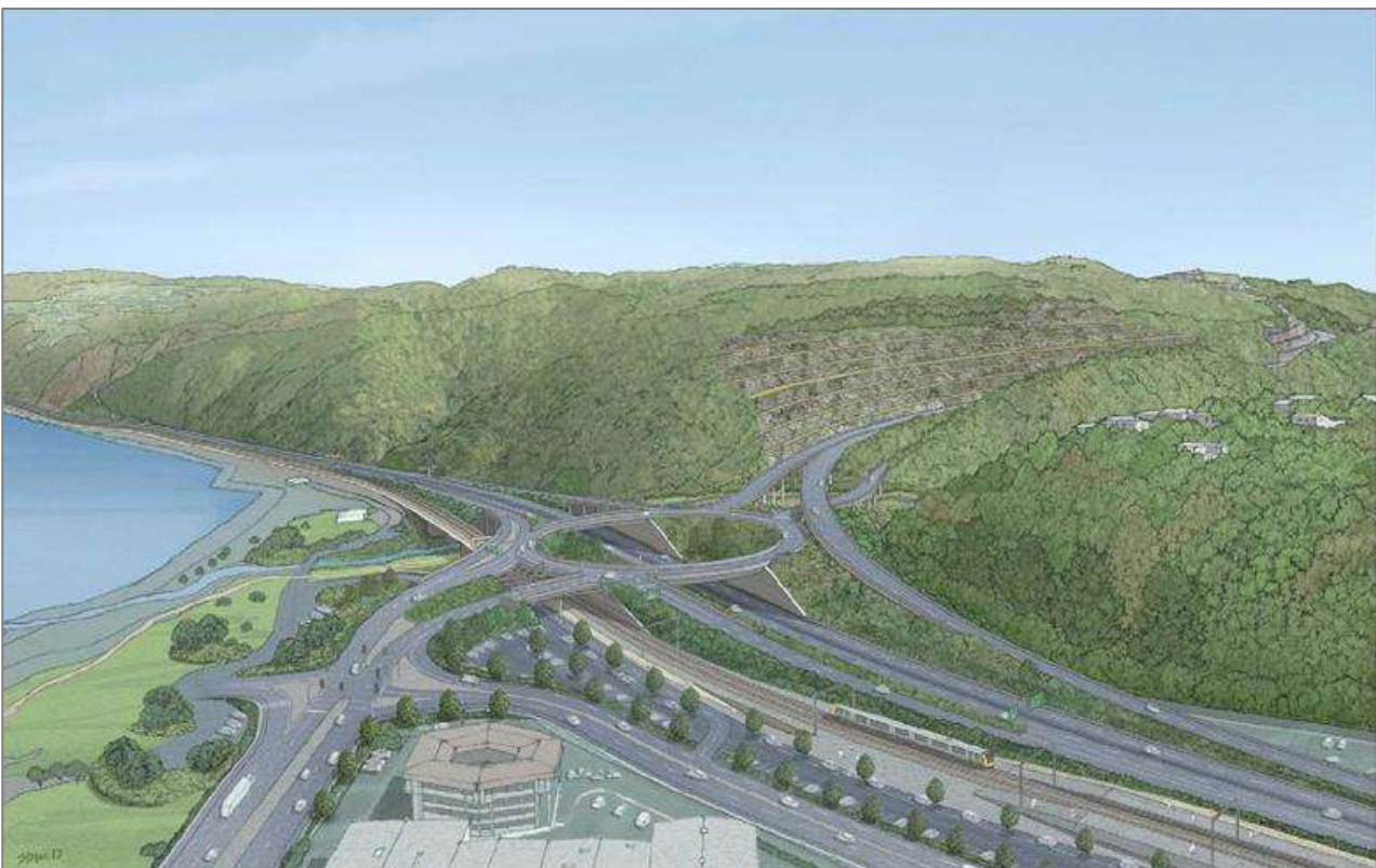
Figure 6 Artist's impression of P2G scheme showing Petone interchange and large Petone cut
