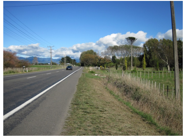
Figure 3-22: Roadside swale adjacent to SH1
