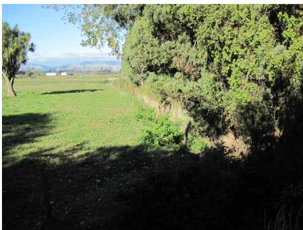
Figure 1-6: Drainage path 3: downstream of Section 3 –south of Paeroa Rd/SH1 intersection
