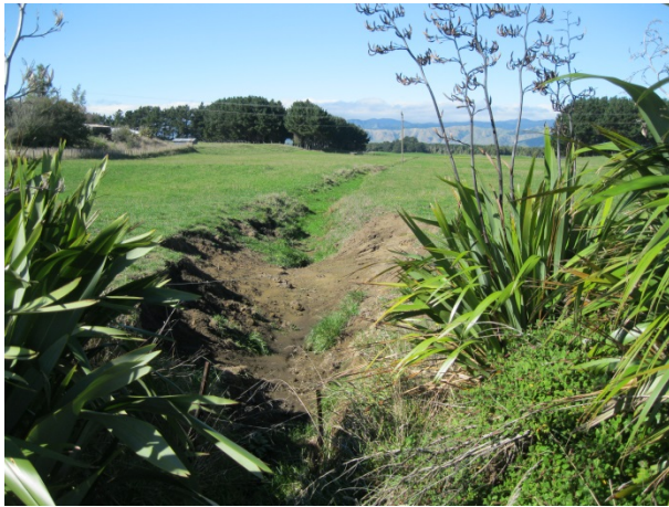
Figure 2-4: Drainage path 1: downstream the road – Section 1 of the project
