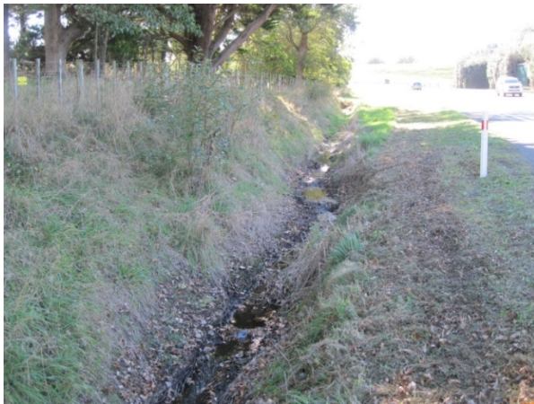
Figure 2-1: Existing road side drainage, SH1
