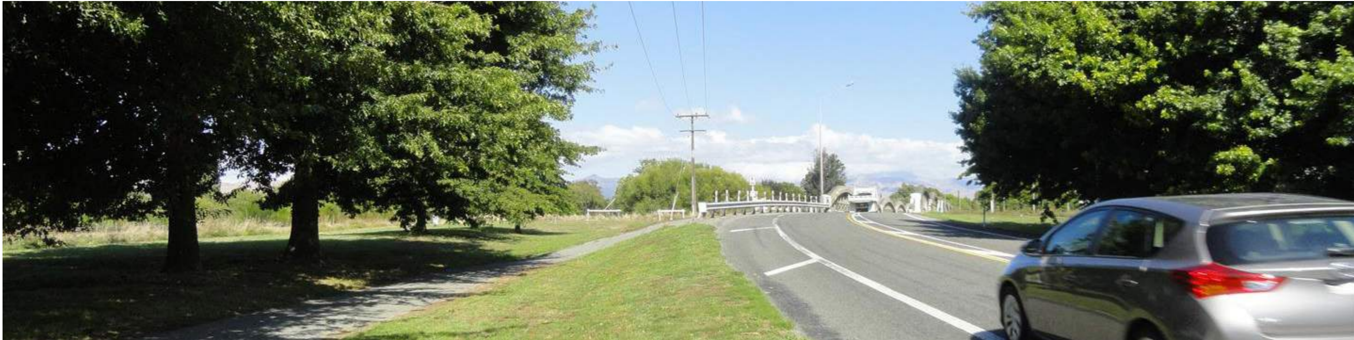
Current Bridge Approach
