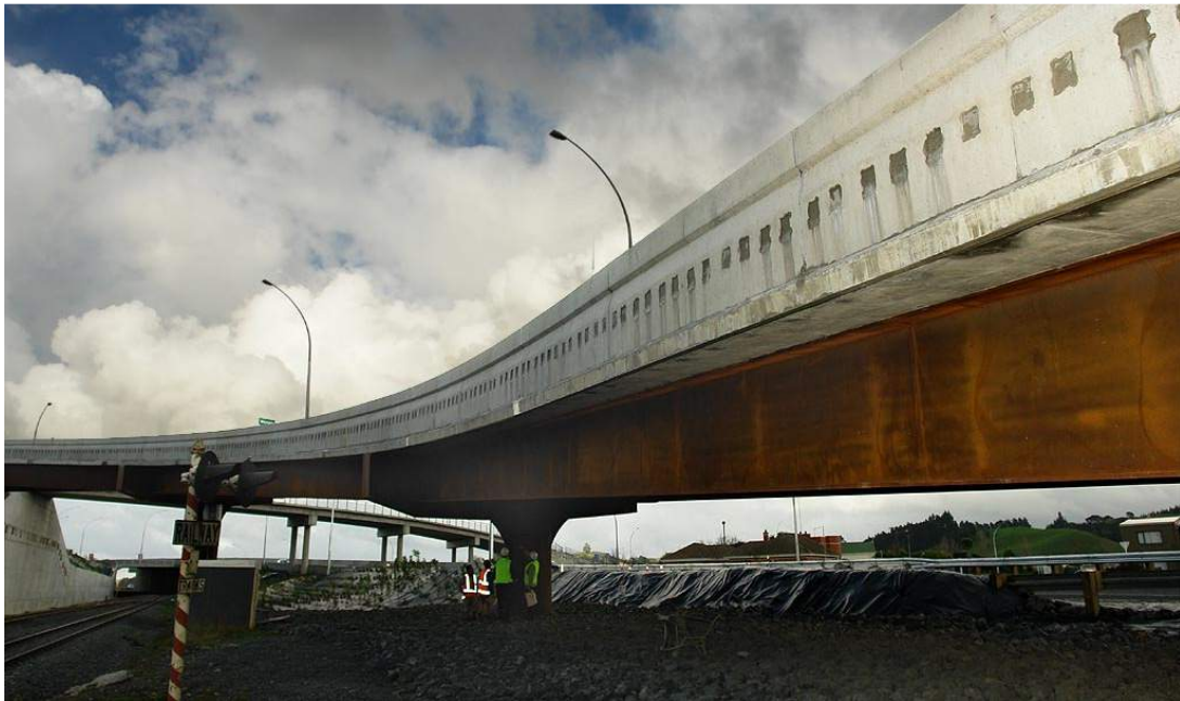
Figure 3.3 SH 1 Mercer Off-ramp
