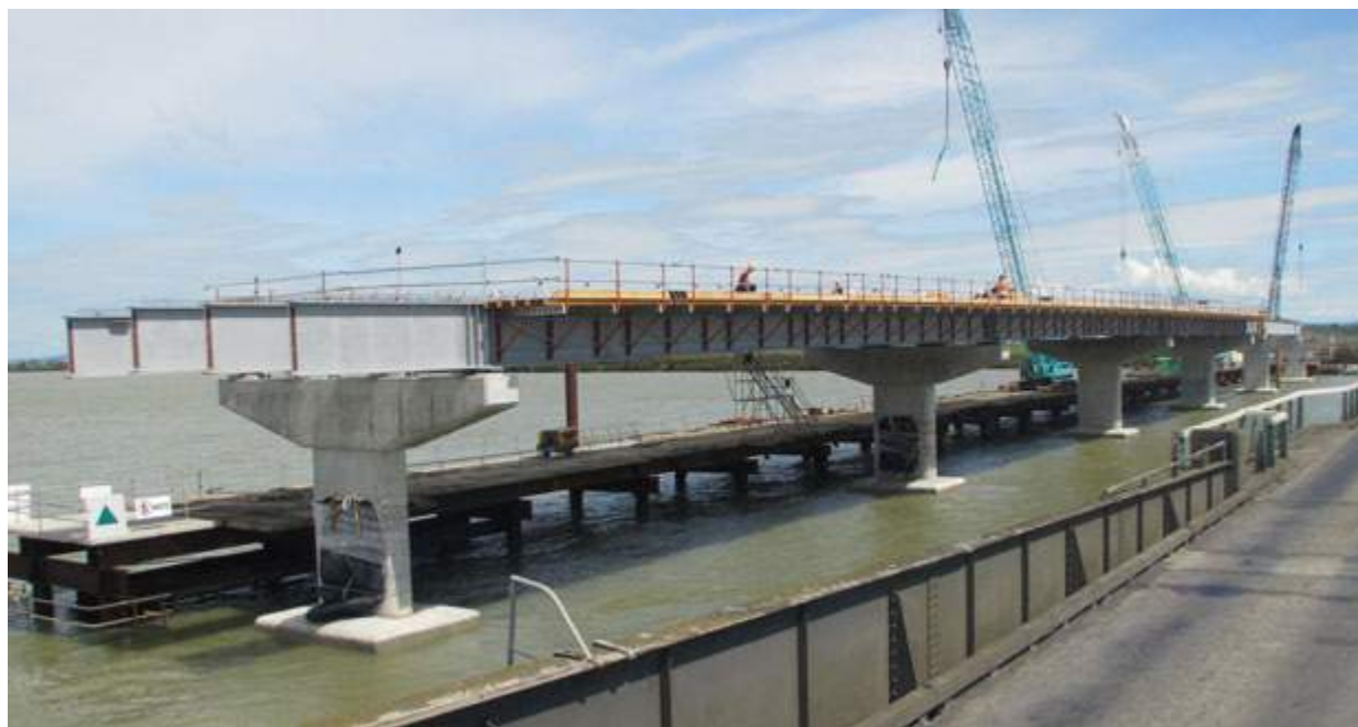
Figure 3.2 SH 25 Kopu Bridge Replacement, Thames
