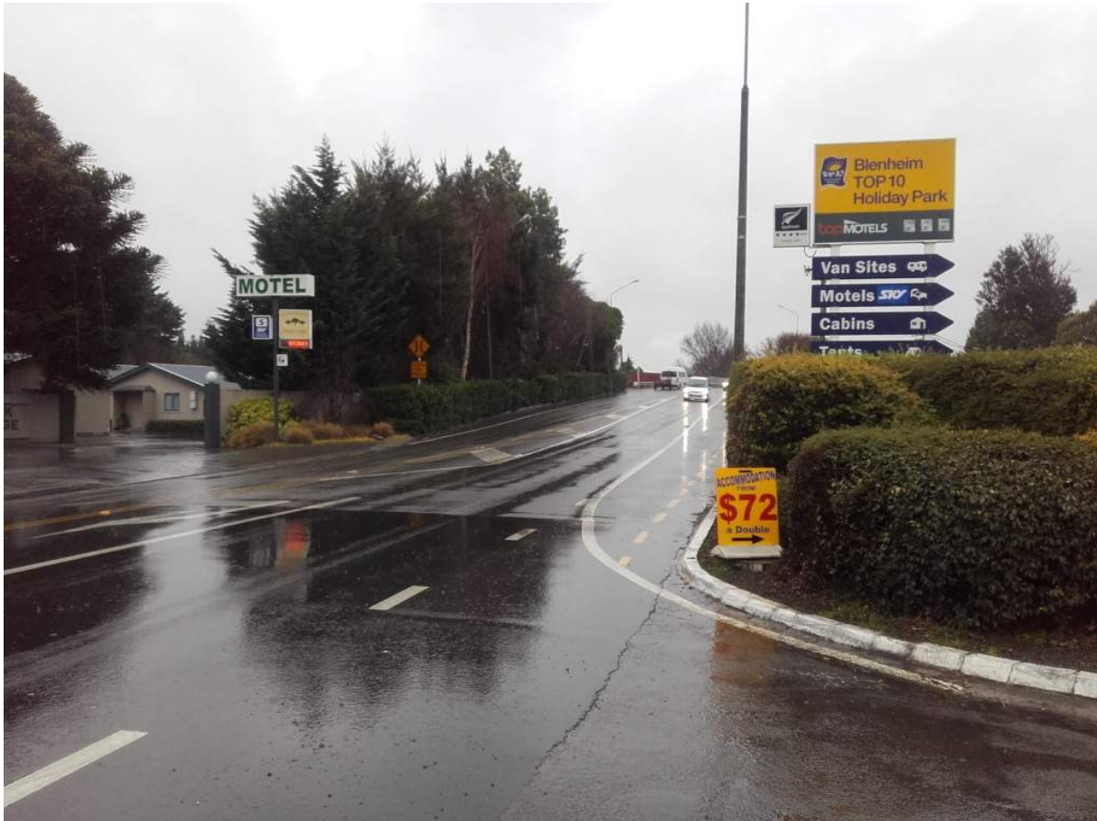
Figure 3 Trees along western property boundary immediately south of Bridge
