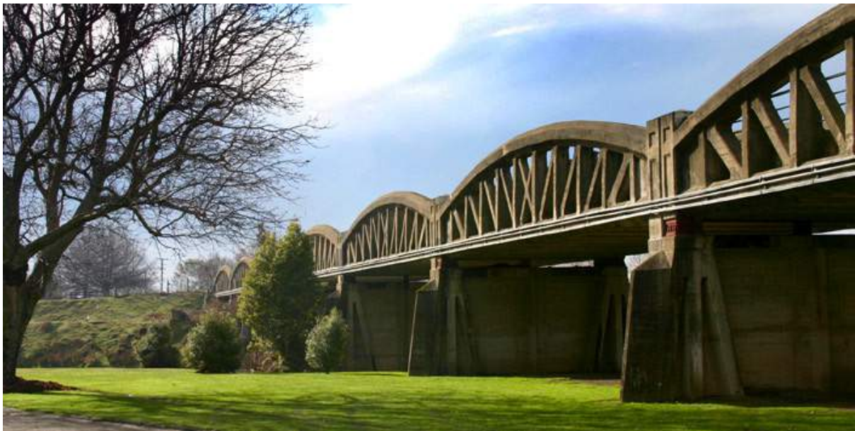
Figure 1.2 – Existing SH1 Opawa River Bridge
