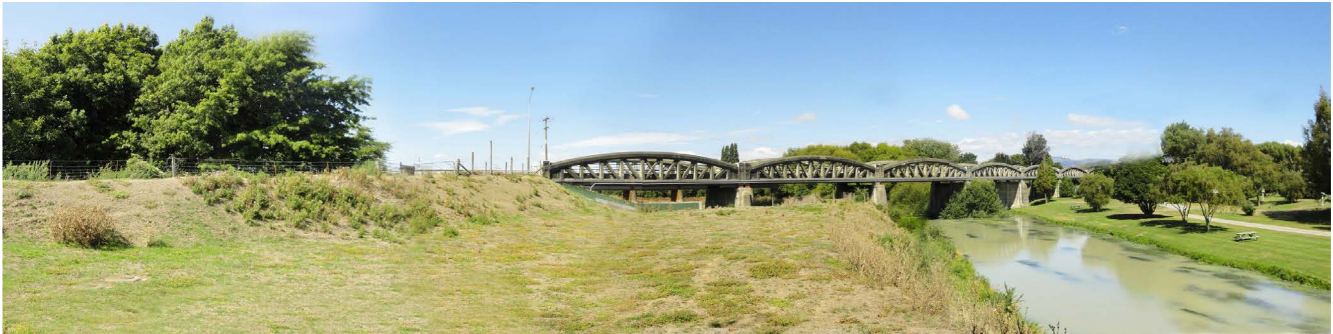
Current View of the Existing Historic Bridge
