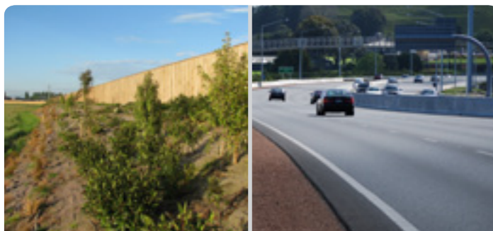
Left: An example of an earth bund with timber acoustic fence on top. Right: An example of a concrete barrier.
