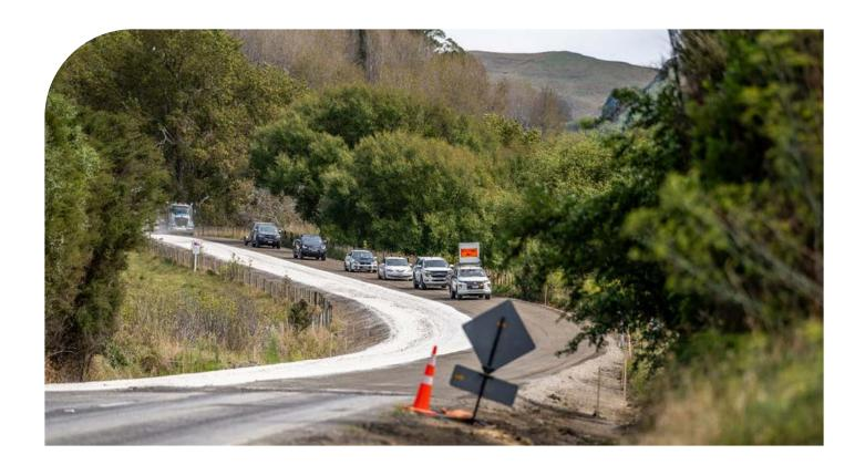
Finally, the pavement was prepared for surfacing, followed by line marking. Following any enabling works a typical site took 8 days to construct
