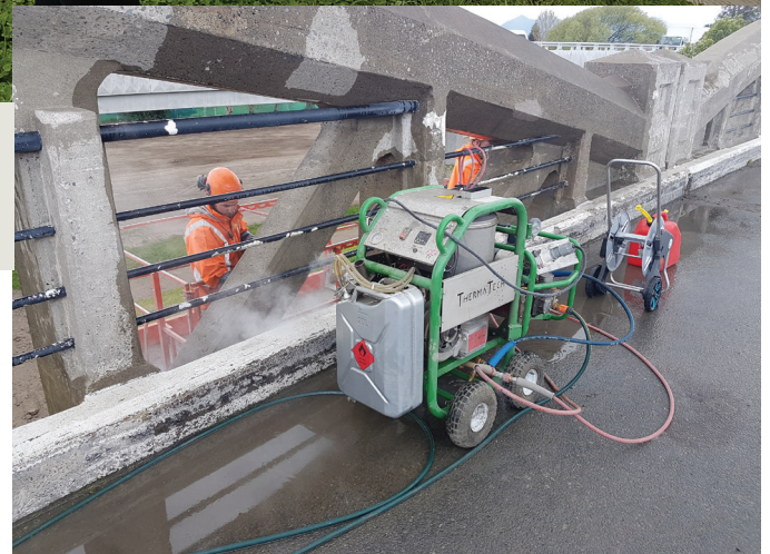
Under Chessa's watchful eye, the old Opawa Bridge is being carefully steam-cleaned.
