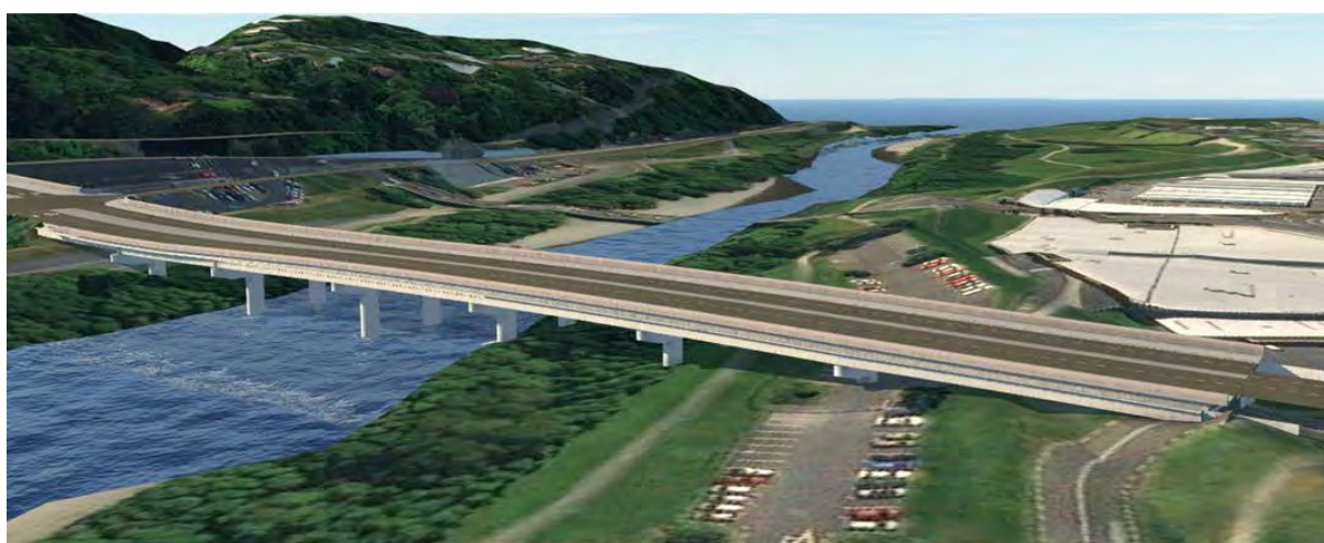
River Bridge: Option 1 – Seven Span Super-T
