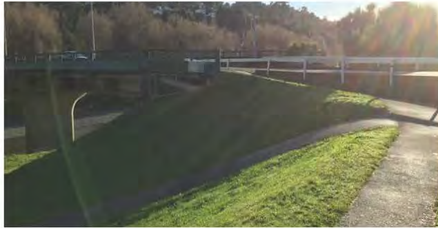
Melling Link Bridge (east abutment)
