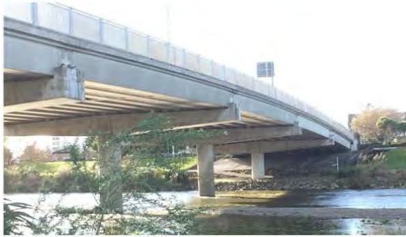
Ewen Bridge (east abutment)
