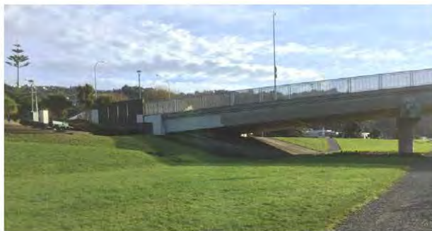
Ewen Bridge (west abutment)
