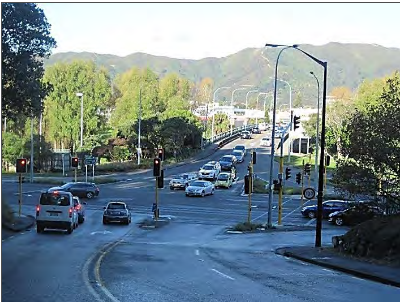
Figure 1: Melling Intersection viewed southeast towards Melling Bridge
