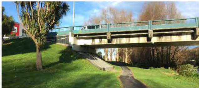
Melling Link Bridge (east abutment)
